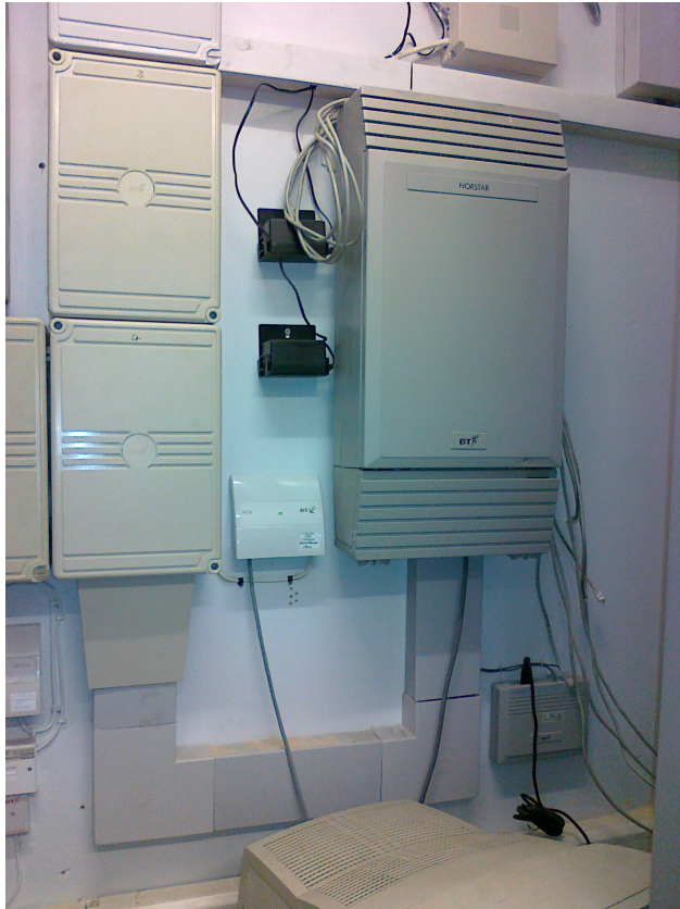
Norstar Modular 0+32 system with wiring boxes on the left
