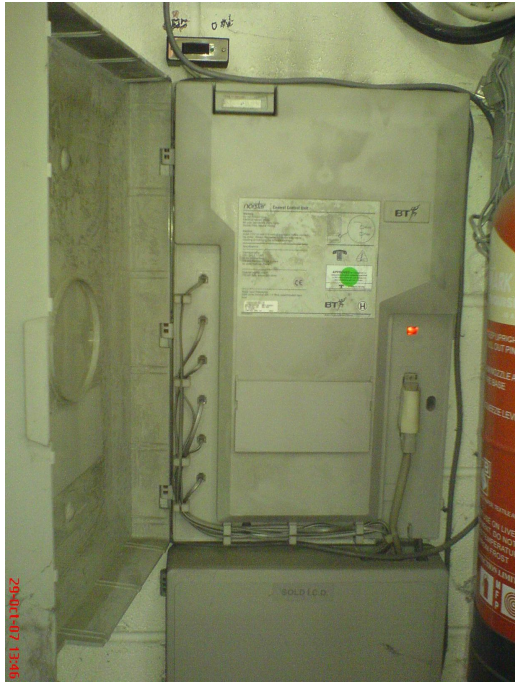
Norstar Compact 6+16 phone system with the power unit and CPU cover opened up
